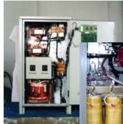
Internal typical view of a three phase AT-OG unit
